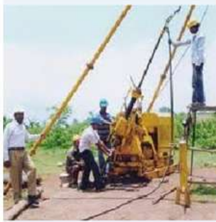
BOREHOLE IN SOIL UNDERWATER WITH LIGHT DUTY CALYEX
