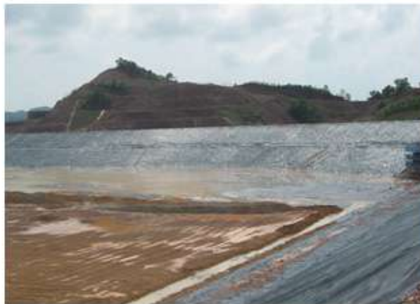
HDPE LINER IN ASH POND ALONG DYKE SLOPES
